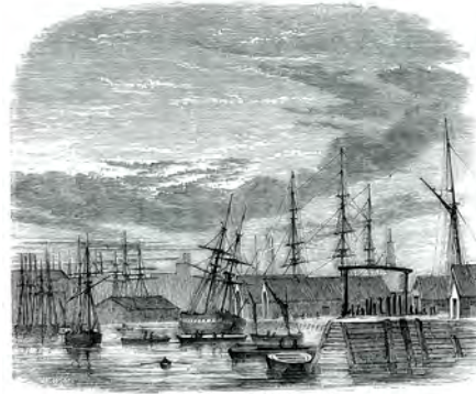
ENTRANCE TO WEST INDIA DOCKS.
