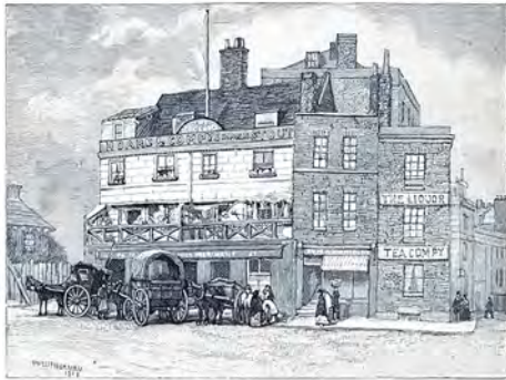
THE OLD GEORGE INN, TOWER HILL.
