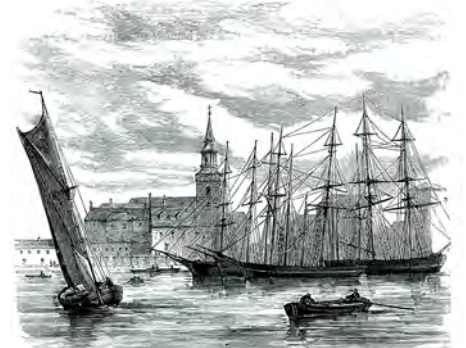
ROTHERHITHE CHURCH: TUNNEL FIER.
