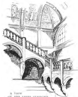
A VIEW ON THE UPPER STAIRCASE. THE IMPERIAL INSTITUTE.
