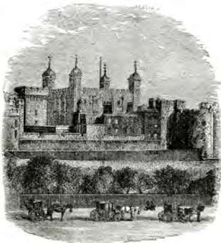
GENERAL VIEW OF THE TOWER.
