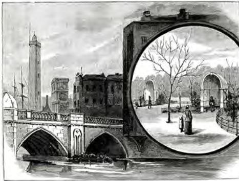
Showing St. Olave's Church and the Shot Tower.
