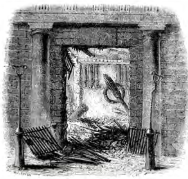
[Entrance, Staircase, &c., of the Great Storehouse after the Fire.]
