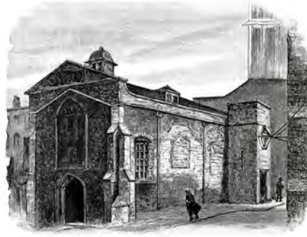
Bell's Chapel, Chancery Lane.
