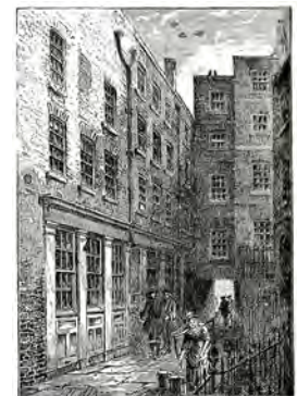
WINE OFFICE COURT, COURT STREET.
