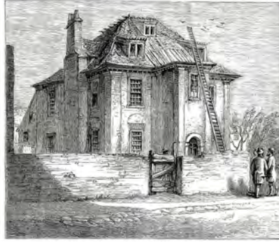
CARR PETER'S HOUSE, HIGBURY FIELDS, ECHELESTON, PULLED DOWN IN JULY 1858.
