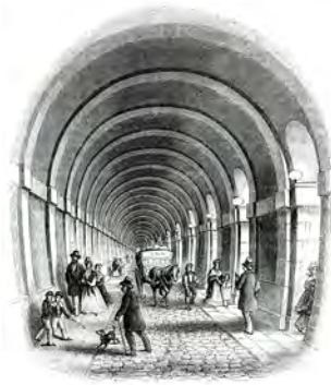
[View to the Tunnel.]
