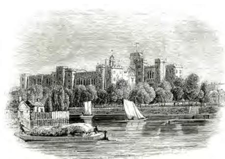
Lambeth Palace, before the recent alterations.
