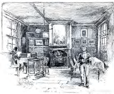
THE CHOP ROOM FIREPLACE.
