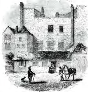
[Exterior of Beauchamp Tower from the Piazza.]
