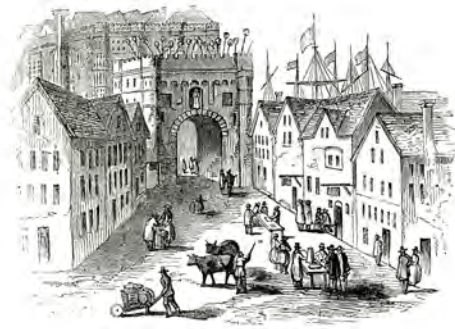
[Approches to London Bridge on the Southwark Side.]
