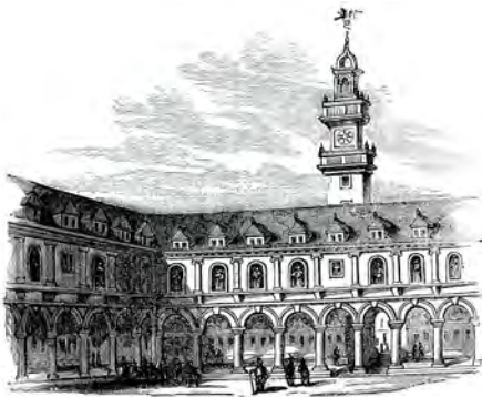
THE ROYAL EXCHANGE, AS BUILT BY GRESHAM.
