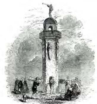
[Conduit in West Cheap.]
