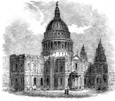
EXTERIOR OF ST. PAUL'S.
