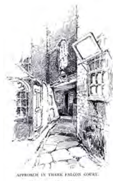
APPROACH IN THESE FRIGON COURT.
