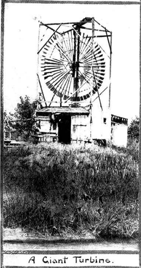
A Simple Turbine Windmill.
