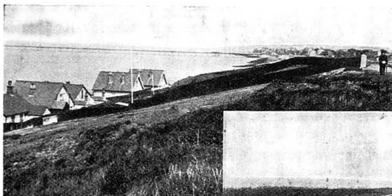
BUNGALOWS LEAD THE WAY.
