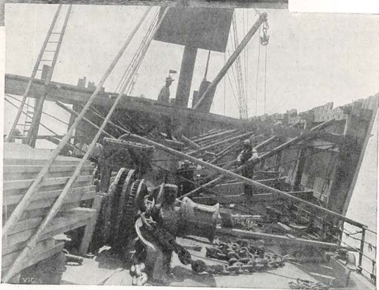
DECK OF "UTOPIA" AFTER RAISING, SHOWING HEAVY NATURE OF COFFERDAM.
