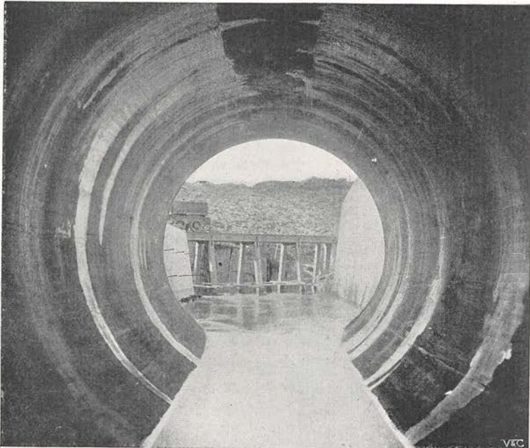
THE BIRMINGHAM WATER SUPPLY: MAKING THE GREAT AQUEDUCT.
