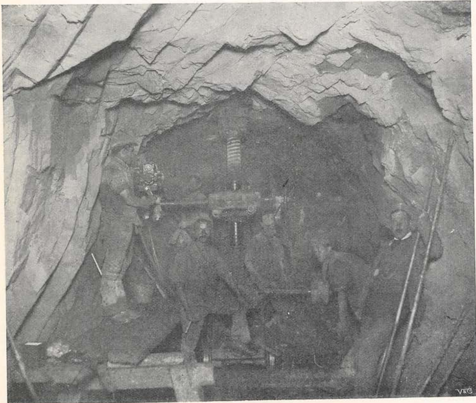
THE BIRMINGHAM WATER SUPPLY: BORING THE AQUEDUCT.
