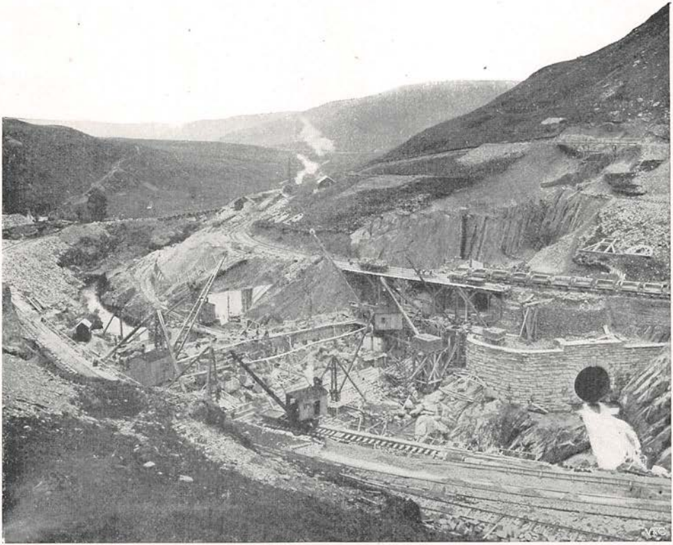
THE BIRMINGHAM WATER SUPPLY : BUILDING THE CRAIG COCH DAM.
