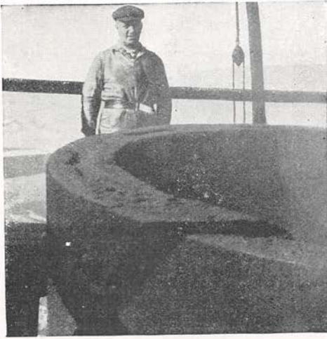
THE LANCASHIRE STEEPLEJACK AT THE SUMMIT OF THE TALLEST CHIMNEY IN ENGLAND, AND—
