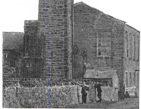
AN UNPROTECTED CHIMNEY THAT WAS STRUCK BY LIGHTNING AND REPAIRED BY MR. SMITH.
