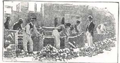
A CLASS IN BRICKLAYING.
