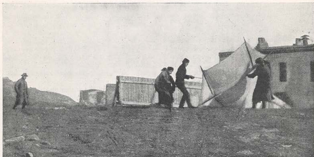
PREPARING TO FLY THE KITE WHICH SUPPORTS THE RECEIVING WIRE. MARCONI ON THE EXTREME LEFT.
