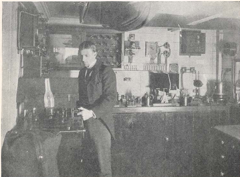
THE ELECTRIC TESTING-ROOM, S.S. "MINIA."
