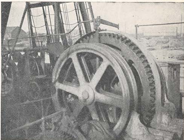
PURCHASE FOR HAULING UP THE CABLE.
