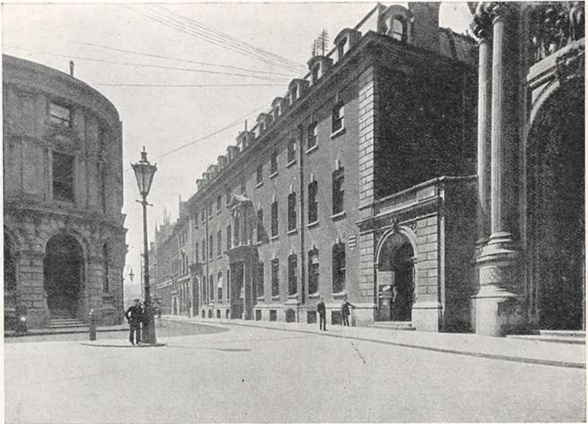
EXTERIOR: BISHOPSGATE STREET END.
