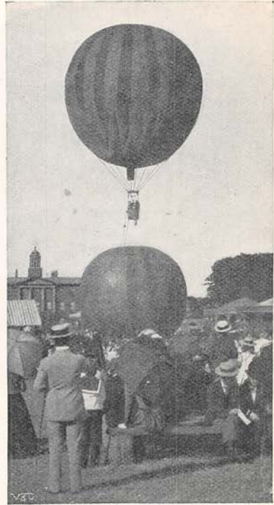
—BUT NO DAMAGE RESULTED.
