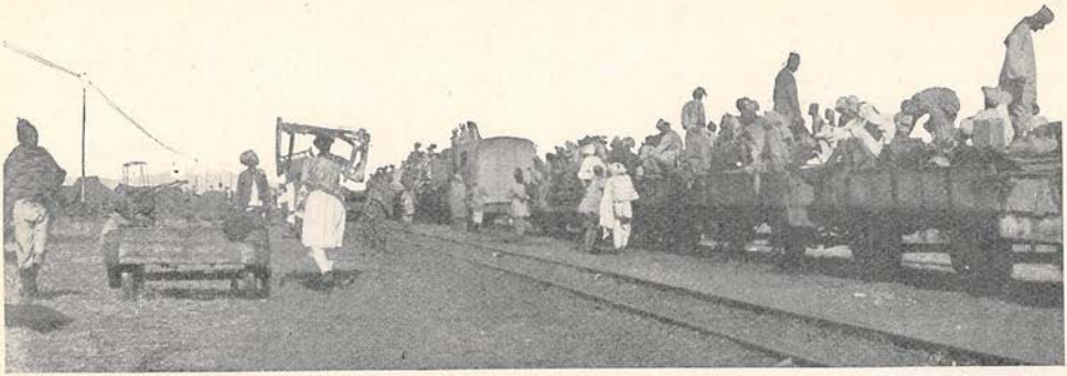
COOLIES' TRAIN WITH MATERIALS AT SULTAN MOHAMED STATION.
