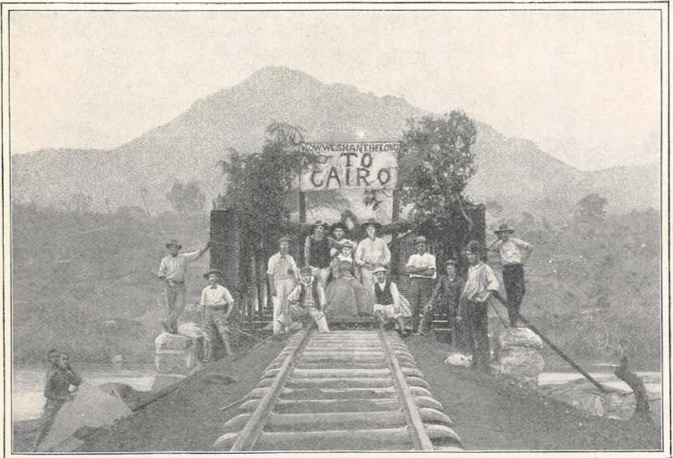
OPENING OF THE IRON RAILROAD BRIDGE ACROSS THE ADZIE RIVER: A RECENTLY COMPLETED PORTION OF THE CAPE TO CAIRO LINE.
