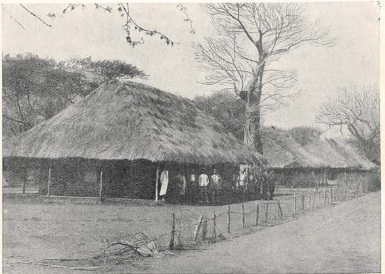
DISTRICT ENGINEER'S OFFICE, KEBWEGI.
