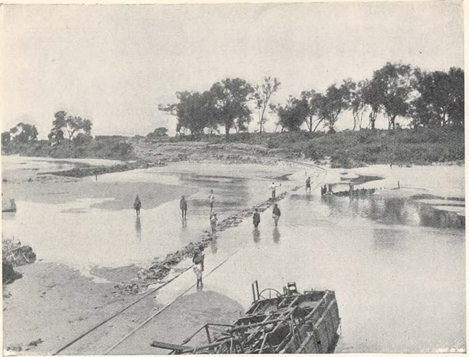
RAILWAY TRACK THROUGH THE SASHI RIVER.
