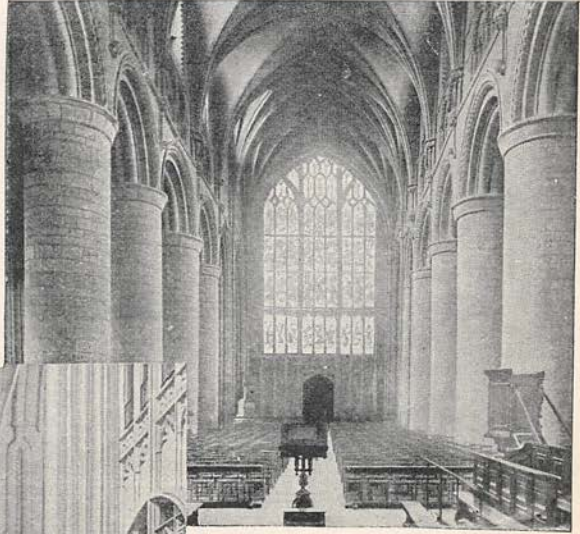
THE NAVE, LOOKING WEST.
