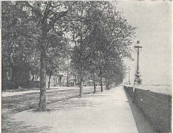
ON THE EMBANKMENT.
