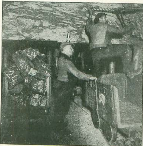
DRILLING THE ROOF OF THE COAL.
