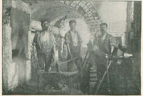
AN UNDERGROUND SMITHY.
