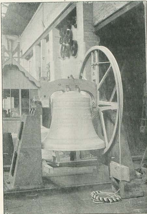
A BELL HUNG TEMPORARILY ON SUPPORTS IN LIEU OF FRAME, TO SHOW WORKING PARTS.
