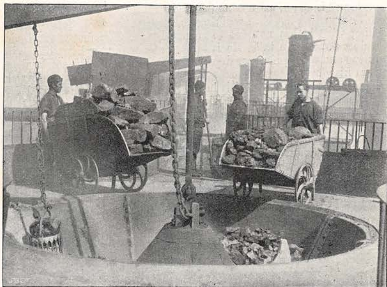
CHARGING WITH COAL AND ORE ON THE TOP OF A FURNACE.
