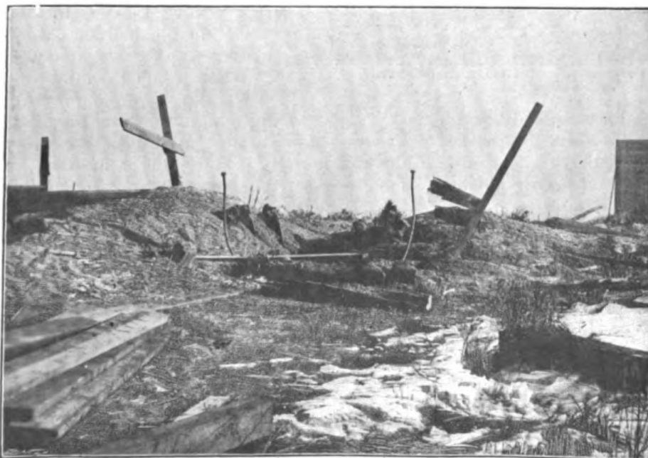
THE COMPLETE DEMOLITION OF THE TARGET AFTER BEING STRUCK BY THE GATHMANN SHELL. From a Photograph.
