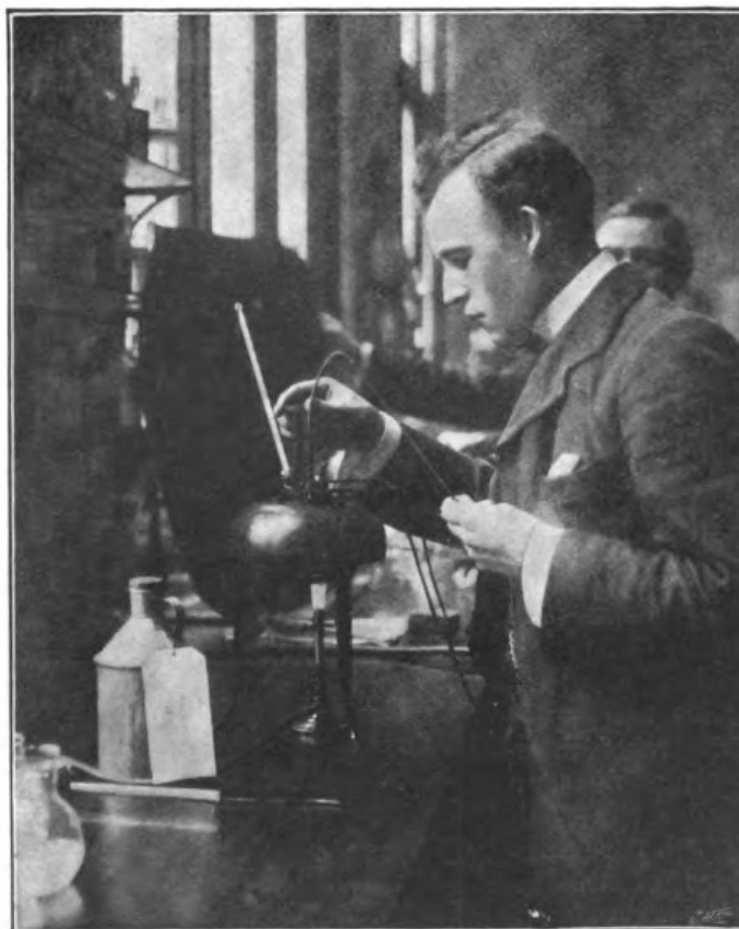
TAKING THE "FLASH-POINT" OF OIL FOR LIGHTHOUSES.
