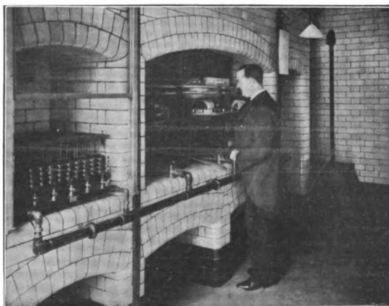
FURNACE FOR INCINERATING TOBACCO.
