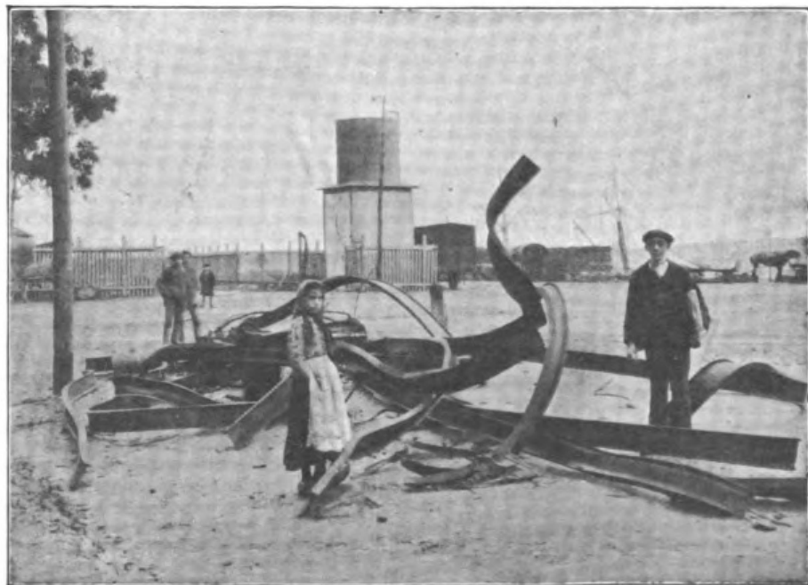
NEAR VIEW SHOWING IRON GIRDERS TWISTED AND CONTOURTED BY THE FORCE OF THE EXPLOSION.
