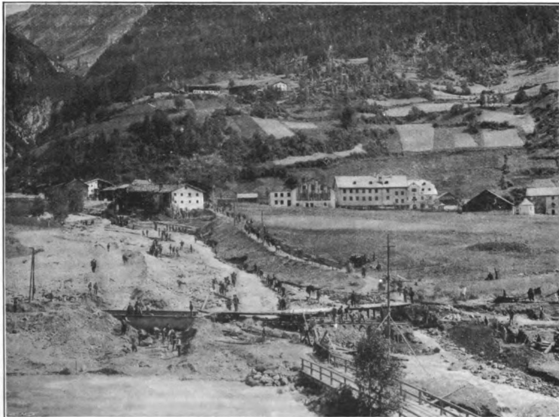
6.—THE LINE AT FLIRSCH WIPED OUT BY AN AVALANCHE. A TEMPORARY TRACK BEING CONSTRUCTED.
