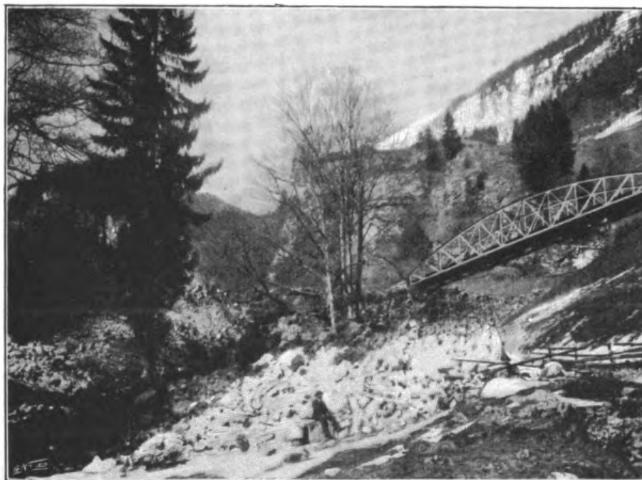
4.—BRIDGE AND LINE DESTROYED BY AN AVALANCHE.
