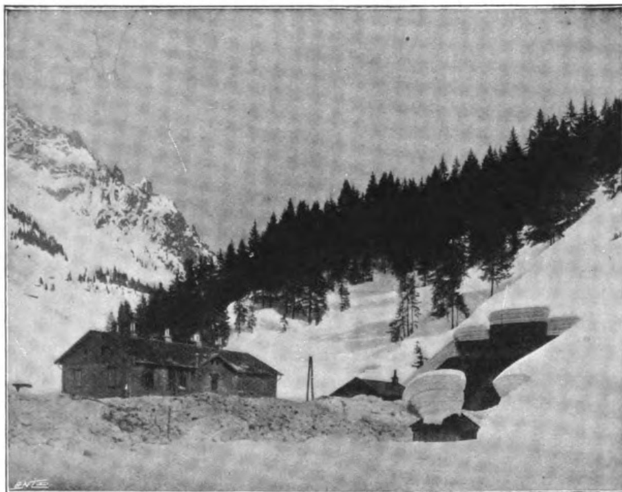
9.—THE MOUTH OF A TUNNEL CLOSED BY AN AVALANCHE.
