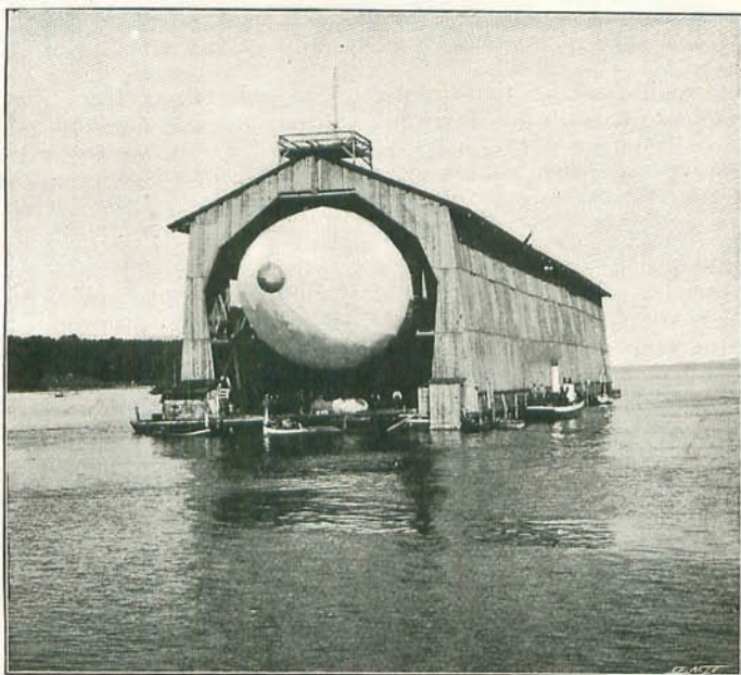
THE ZEPPELIN AIR-SHIP IN ITS FLOATING HOUSE ON LAKE CONSTANCE—SHOWING THE REAR END, WHICH IS CONICAL IN SHAPE.
