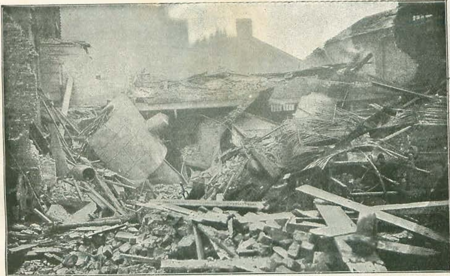
THE EXPLOSION AT ASHLEY LANE, MANCHESTER, DECEMBER 23, 1867.
