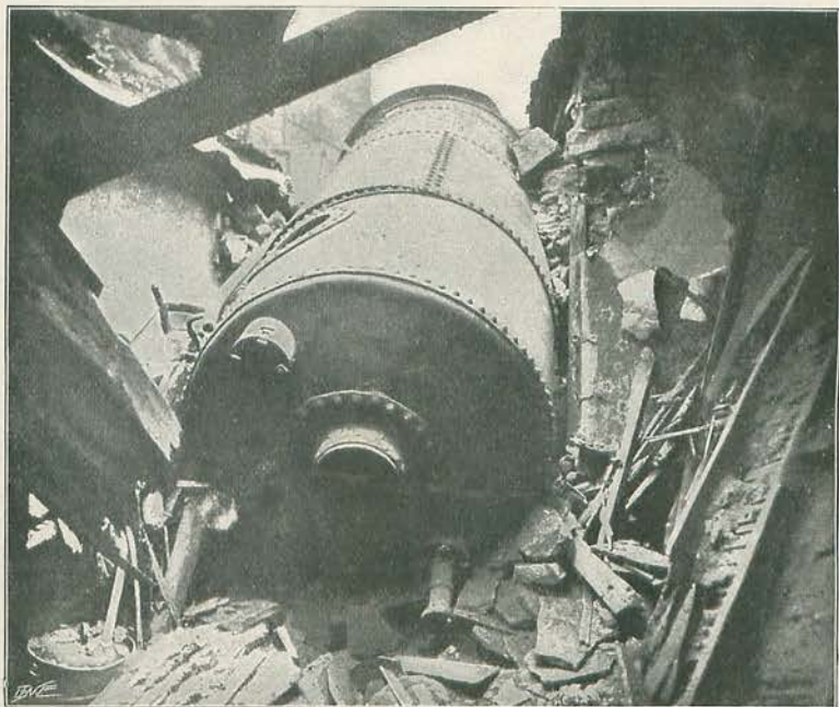
THE BURNLEY EXPLOSION, MARCH 4, 1892. THE BOILER LYING IN AN UPPER ROOM OF "THE CROSS KEYS INN," HAVING ENTERED THROUGH THE ROOF.
