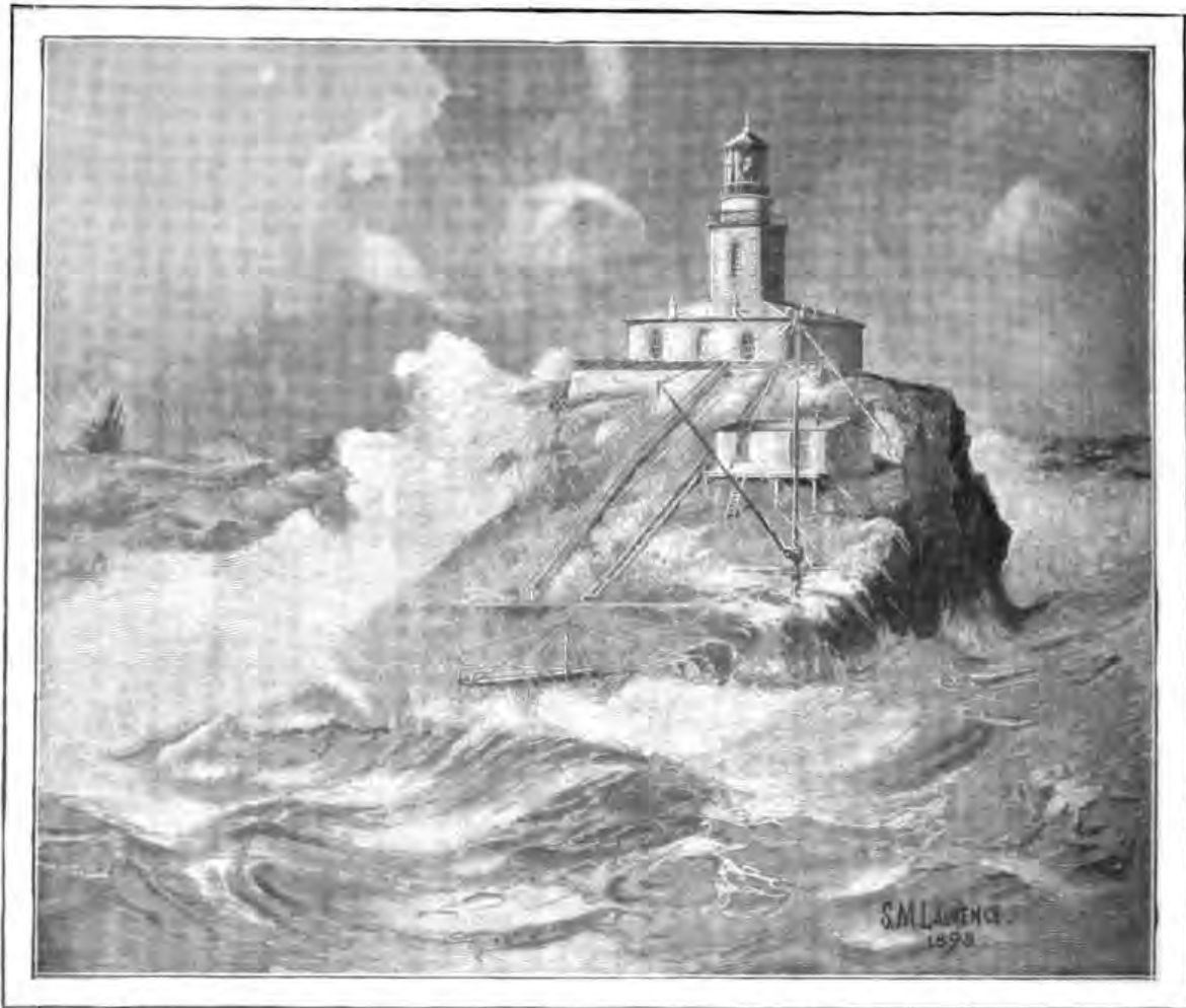
A STORM AT THE TILLAMOOK ROCK LIGHTHOUSE, OREGON.
