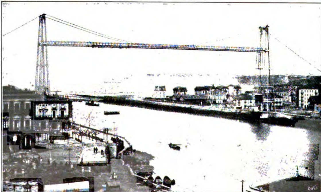
GENERAL VIEW OF THE PORTUGUESE FERRY BRIDGE OVER THE NERVION.
