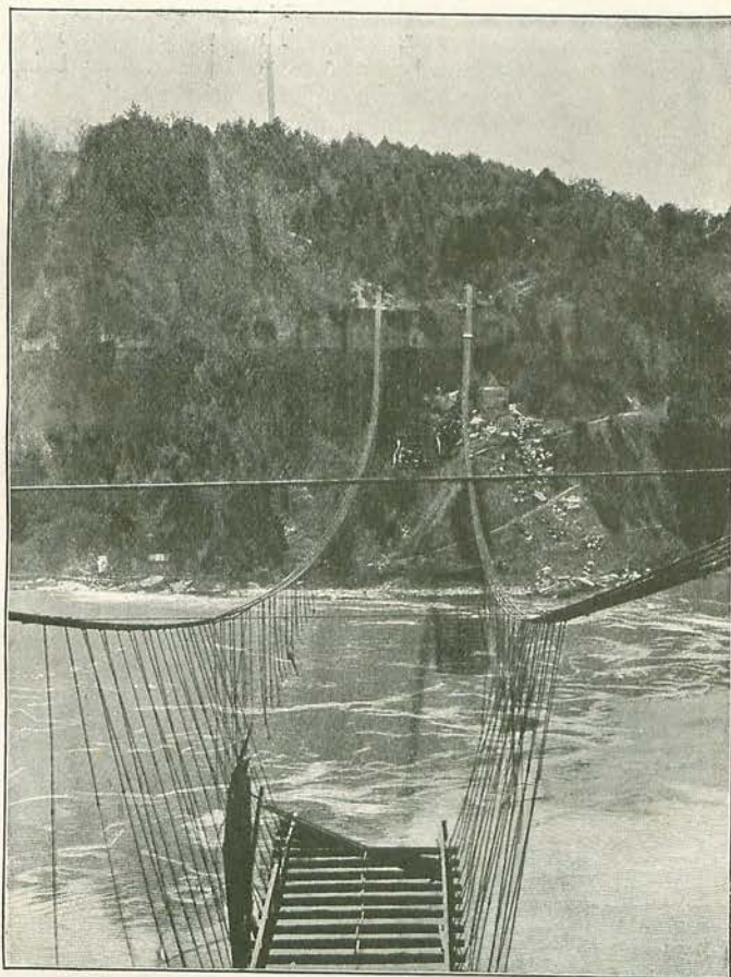
14.—WRECK OF THE SECOND SUSPENSION BRIDGE, FEBRUARY 1, 1864—SHOWING From a] THE CABLES OVER WHICH THE CRIMINALS ESCAPED. [Photograph.
