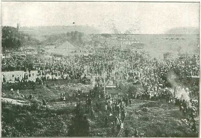
7.—CELEBRATION OF THE COMPLETION OF THE FIRST ARCH BRIDGE—NEW YORK SIDE.
