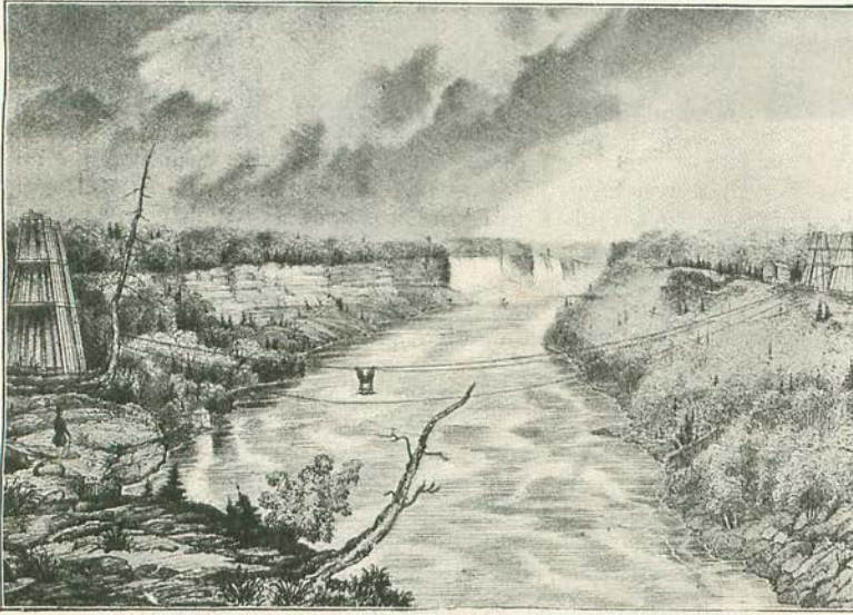
2.—THE FIRST CABLEWAY—ON THE SITE OF THE FIRST SUSPENSION BRIDGE. From an Old Print.
