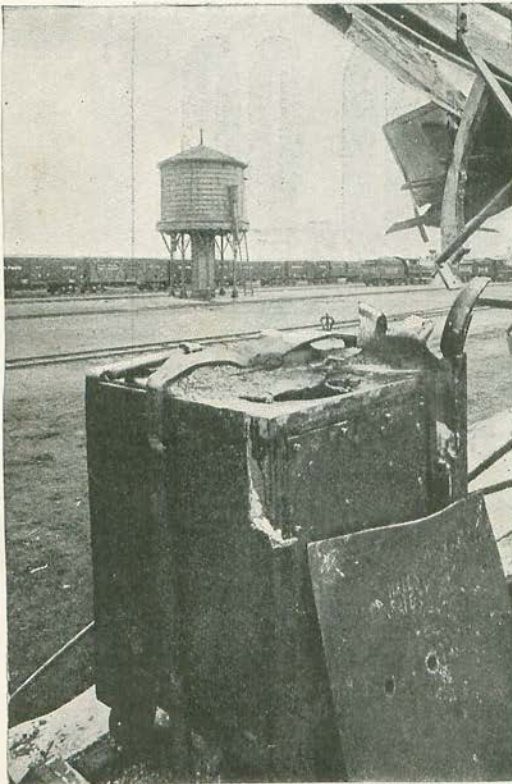
TOP VIEW OF SAFE.
