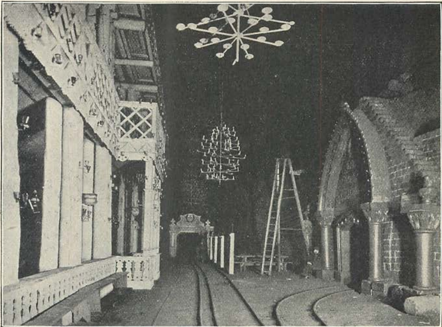
THE RAILWAY STATION ON THE THIRD FLOOR.
