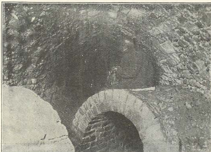
NATURAL CAVE, THROUGH WHICH BUCKLETSBURY SEWER IS CUT.
