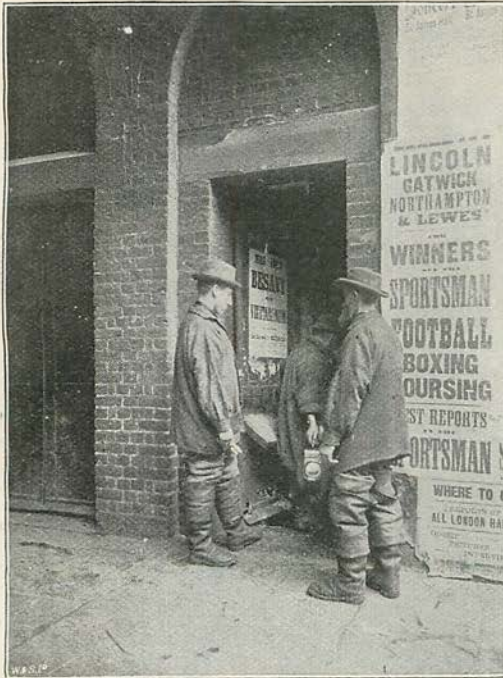
ENTRANCE IN SHOE LANE TO THE SUBWAY SEWERS.
