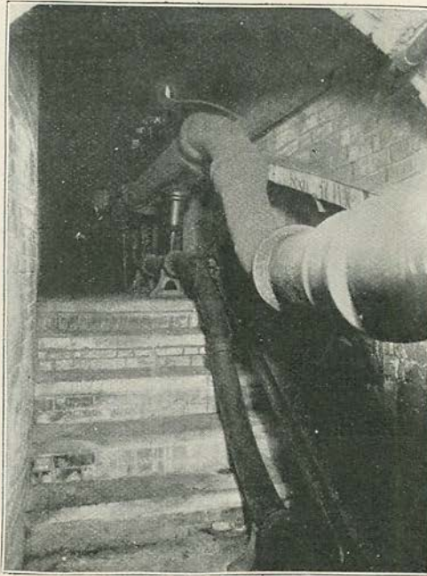
A NARROW SUBWAY OVER THE L. C. AND D. RAILWAY.
