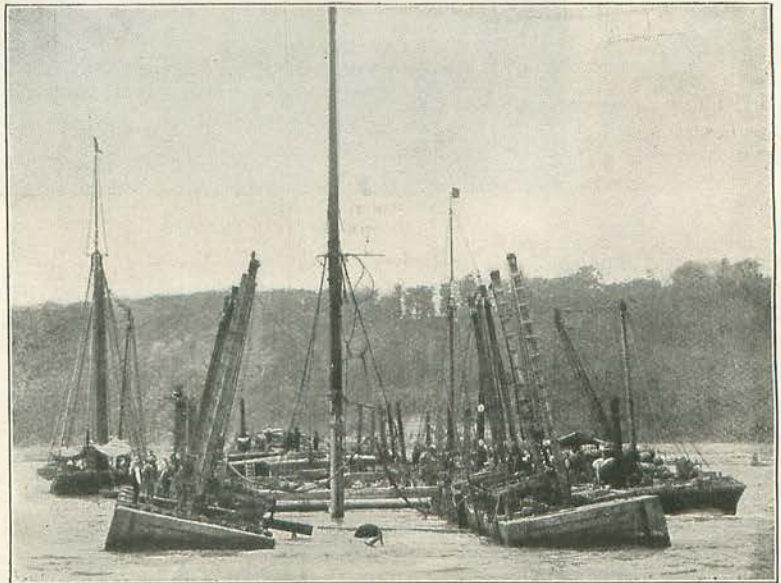
SHOWING HOW THE "WELLS CITY" WAS LIFTED.
