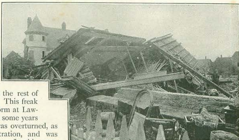
HOUSE WRECKED AND PIANO OVERTURNED AT LAWRENCE, MASS.
