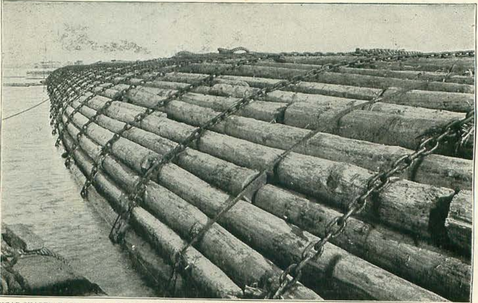
CIGAR-SHAPED RAFT BUILT ON THE PACIFIC COAST. LENGTH 528FT., CONTAINING 560,000 LINEAL FEET OF TIMBER. Photo. from the Pacific Illustrating Bureau, San Fran., Cal.
