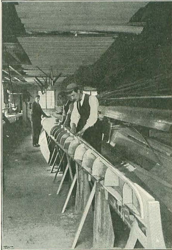
SECOND STAGE—THE BOAT PARTIALLY PLANKED, THE SHELL NOW ALMOST COMPLETE.
