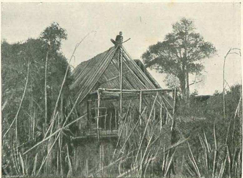
BUILDING NEWALA CHURCH.
