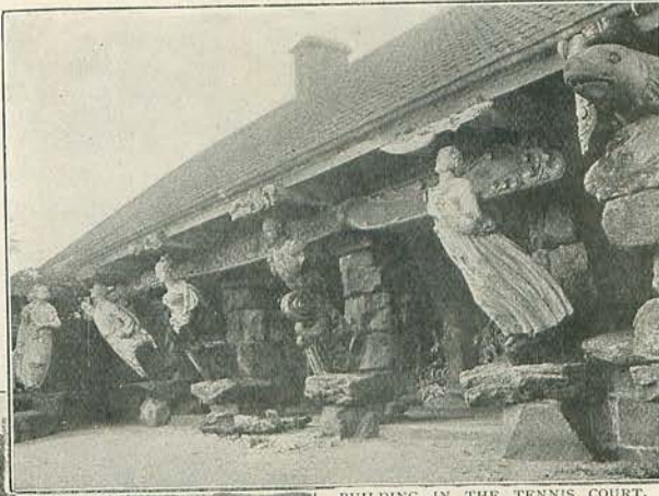
BUILDING IN THE TENNIS COURT. From a Photo. by C. J. King, Scilly.
