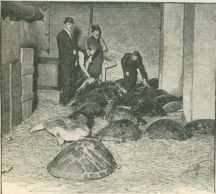
INTERIOR OF MR. BELLIS'S TURTLE WAREHOUSE.
