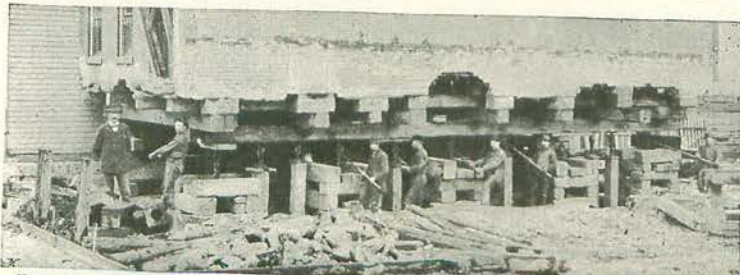
LIFTING THE ABOVE HOUSE BY MEANS OF JACK-SCREWS.
