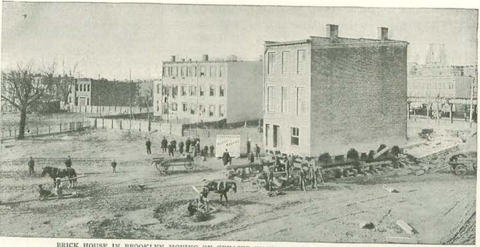
BRICK HOUSE IN BROOKLYN MOVING ON GREASED WAYS—HORSES AND CAPSTANS AT LEFT. From a Photograph.
