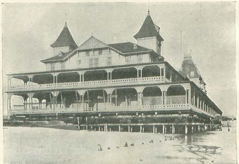
MOVING THE BRIGHTON BEACH HOTEL, IN 1888, AWAY FROM THE ENCREACHING ATLANTIC—SHOWING THE TRUCKS UNDER THE HOTEL. [J. H. Beal, New York City.
