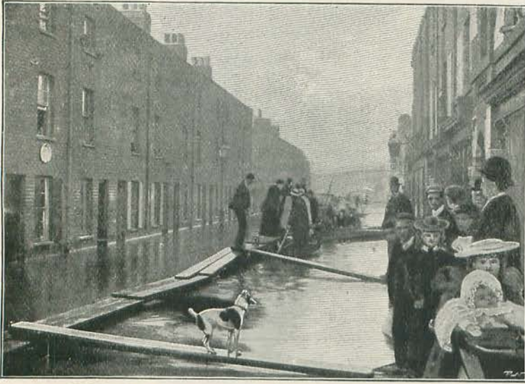
7.—OXFORD ROAD, ETON, DURING THE THAMES FLOODS OF NOVEMBER, 1894. From a Photo. lent by G. J. Symons, Esq.
