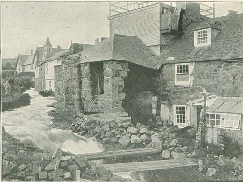
13.—HOUSE AT ST. IVES WASHED DOWN BY FLOODS. From a Photo. by J. C. Burrow, Camborne.
