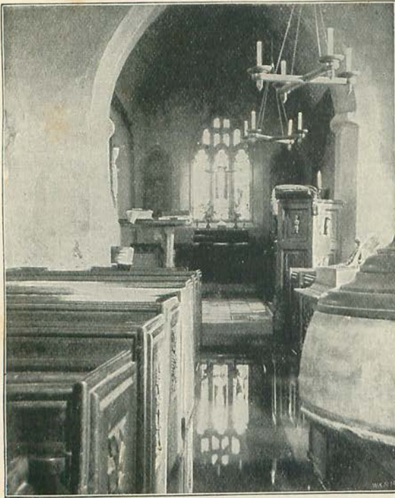
15.—FLOODED FLOOR IN MILSTON CHURCH, NEAR AMESBURY. From a Photo. lent by G. J. Symons, Esq.
