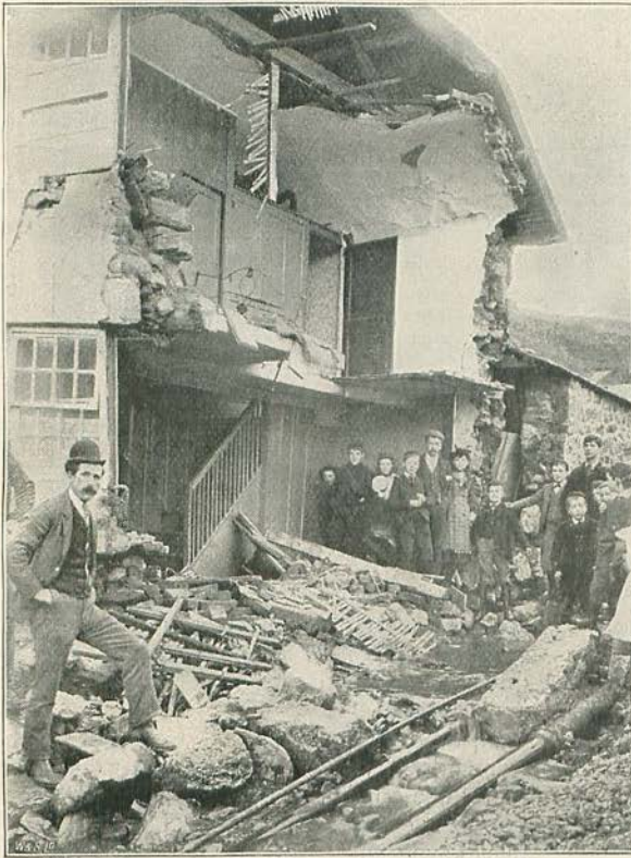
11.—HOUSE AT ST. IVES, DEMOLISHED BY FLOODS. From a Photo. by J. C. Burrow, Camborne.
