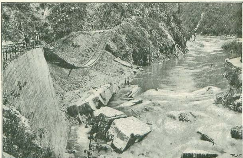
2.—PART OF THE RAILWAY IN JAMAICA UNDERMINED BY FLOODS. From a Photo. lent by the Costa Rica Railway Co.
