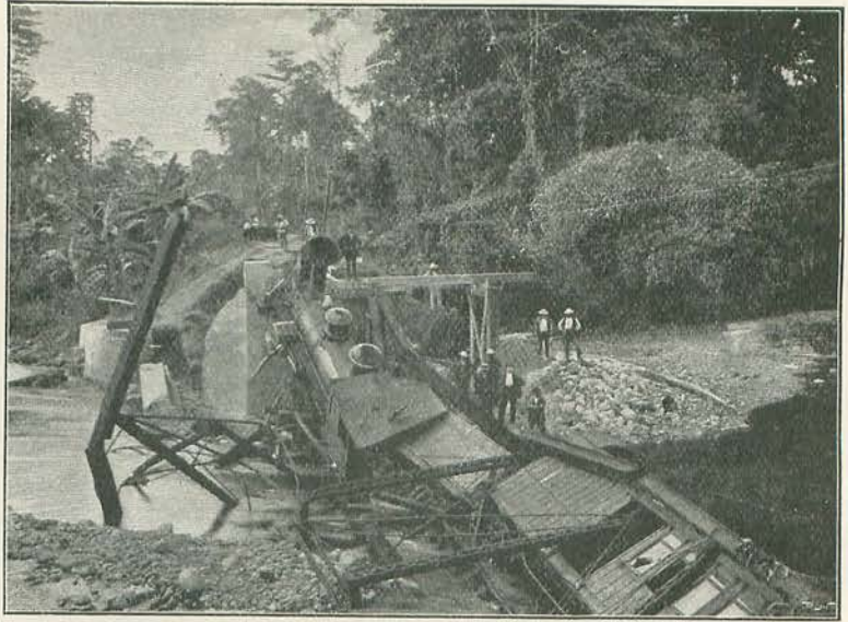
4.—TRAIN AND BRIDGE DEMOLISHED BY FLOODS ON THE COSTA RICA RAILWAY. From a Photograph.
