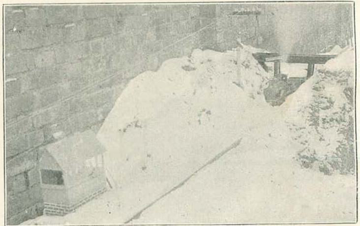
4.—SIGNAL CABIN, AND SNOW-FILLED CUTTING.
