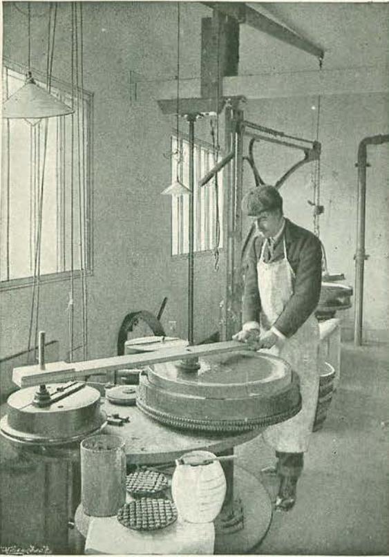
POLISHING AN OBJECT-GLASS. From a Photo. by Sir Howard Grubb.
