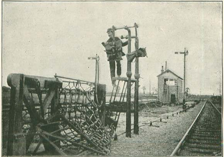
FIG. 4.—TURNING THE STANDARDS INTO POSITION.
