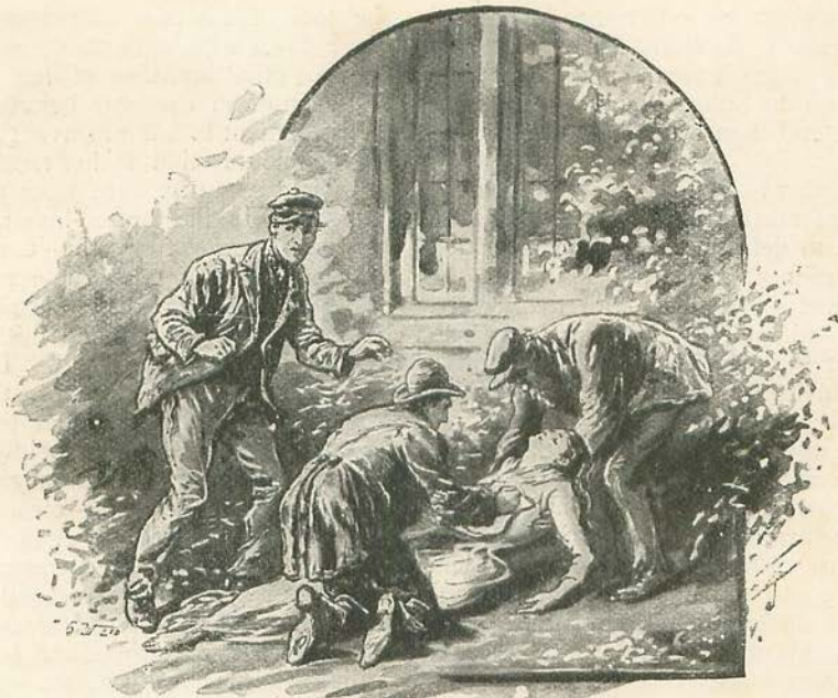
"THEY LAID HER IN FRONT OF THE WINDOWS."
