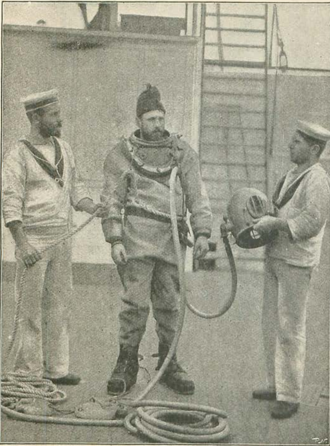
DIVER ON BOARD H.M.S. "CAMPERDOWN" DRESSING TO REPAIR THE BREACH.
