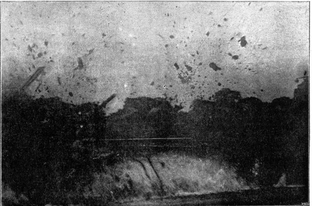
FIG. 17.—BLOWING UP DOCK WALL, NEWPORT, BY DYNAMITE.
