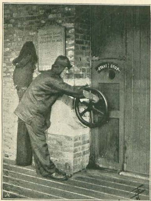
NO. 8.—STARTING THE INCORPORATING MILL.
