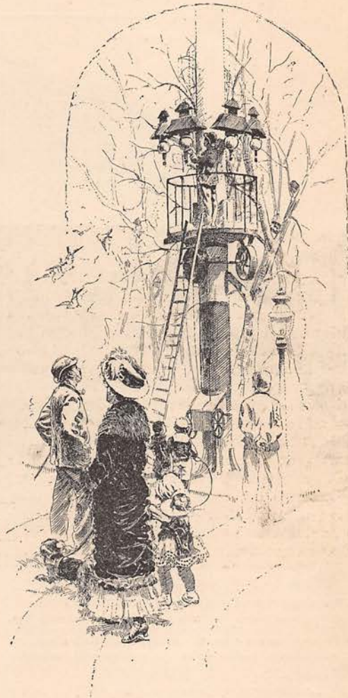
THE LAMPS LOWERED. FITTING-IN THE NEW RODS.
