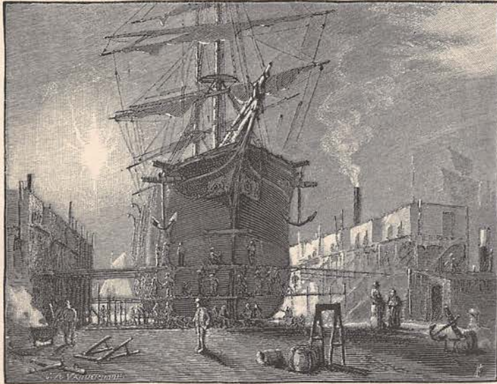
A SECTIONAL DOCK.
