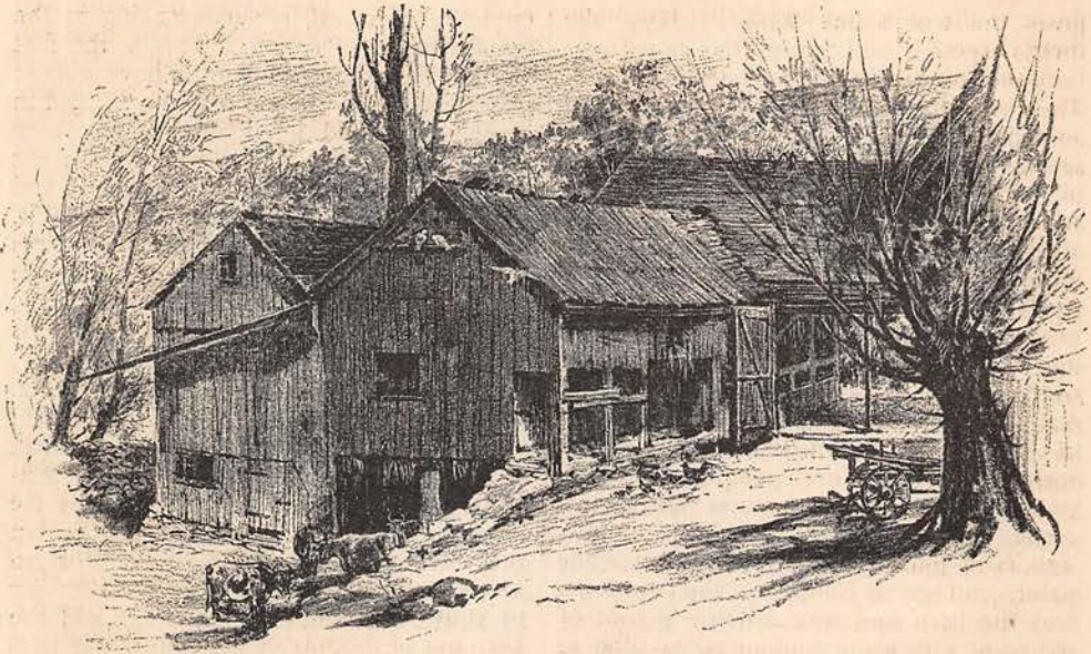
Old barn with cattle sheds
