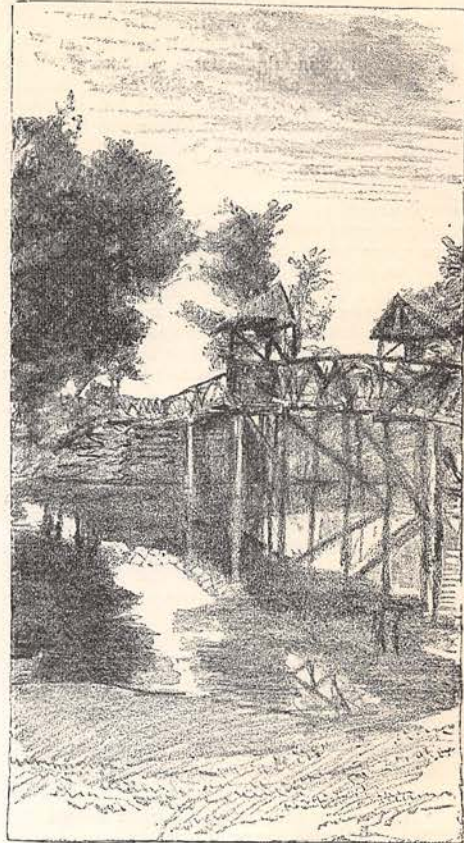
THE OLD NORTH BRIDGE REBUILT.
