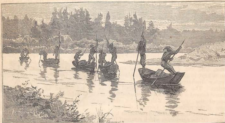
POLING UP THE STONES FOR THE GATE-WAY.
